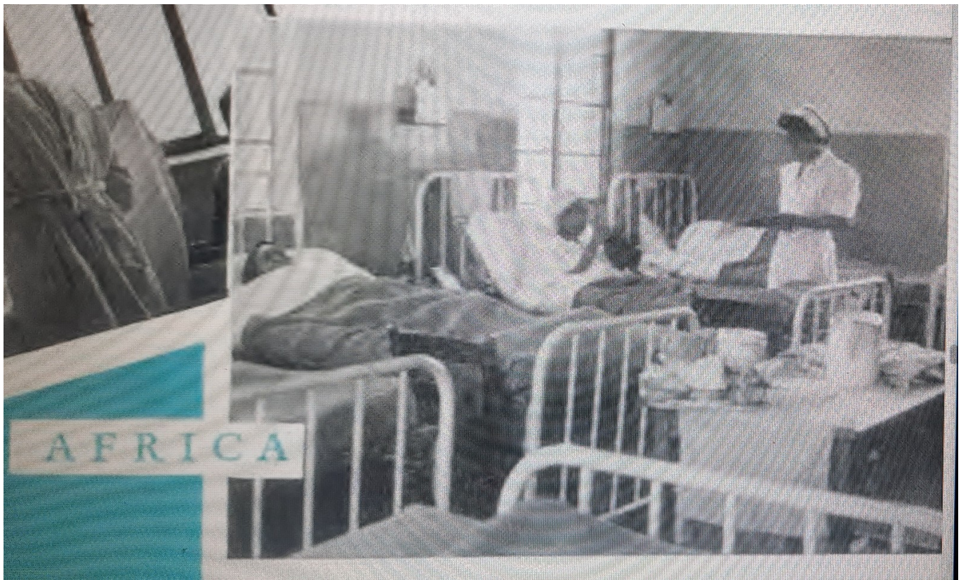
Nokuphila Hospital showing inside a ward.
