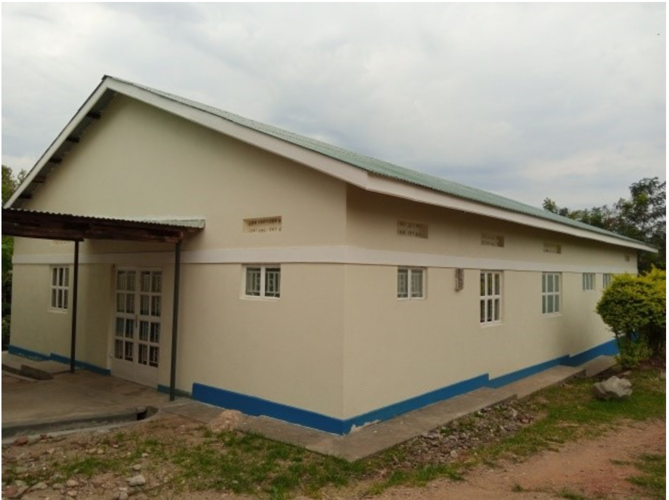
Ebenezer SDA Health Centre operating theatre.
