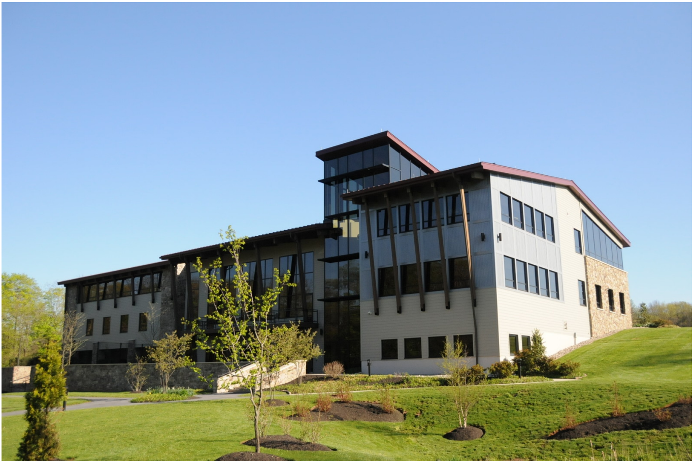
Allegheny East Conference headquarters building
