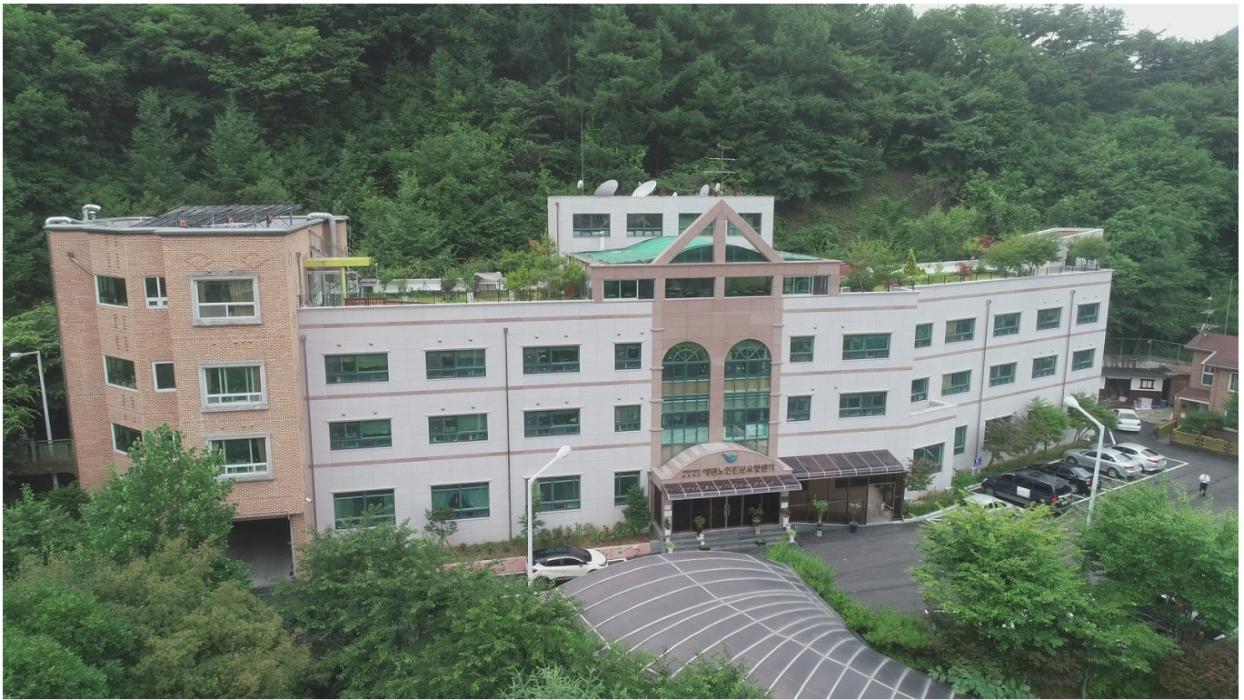
Main building of the Eden Senior Sanitarium Center Photo courtesy of Eden Senior Sanitarium Center.
