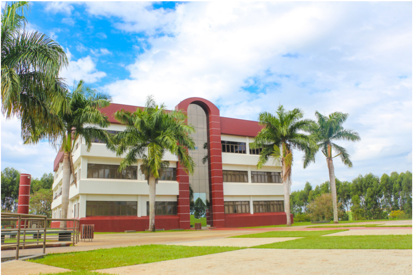
College building facade in 2017
