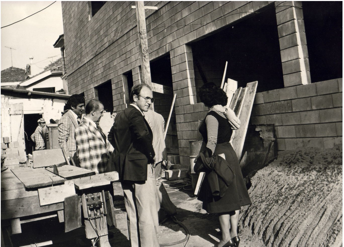
Construction of Varzea Grande Adventist Academy.
